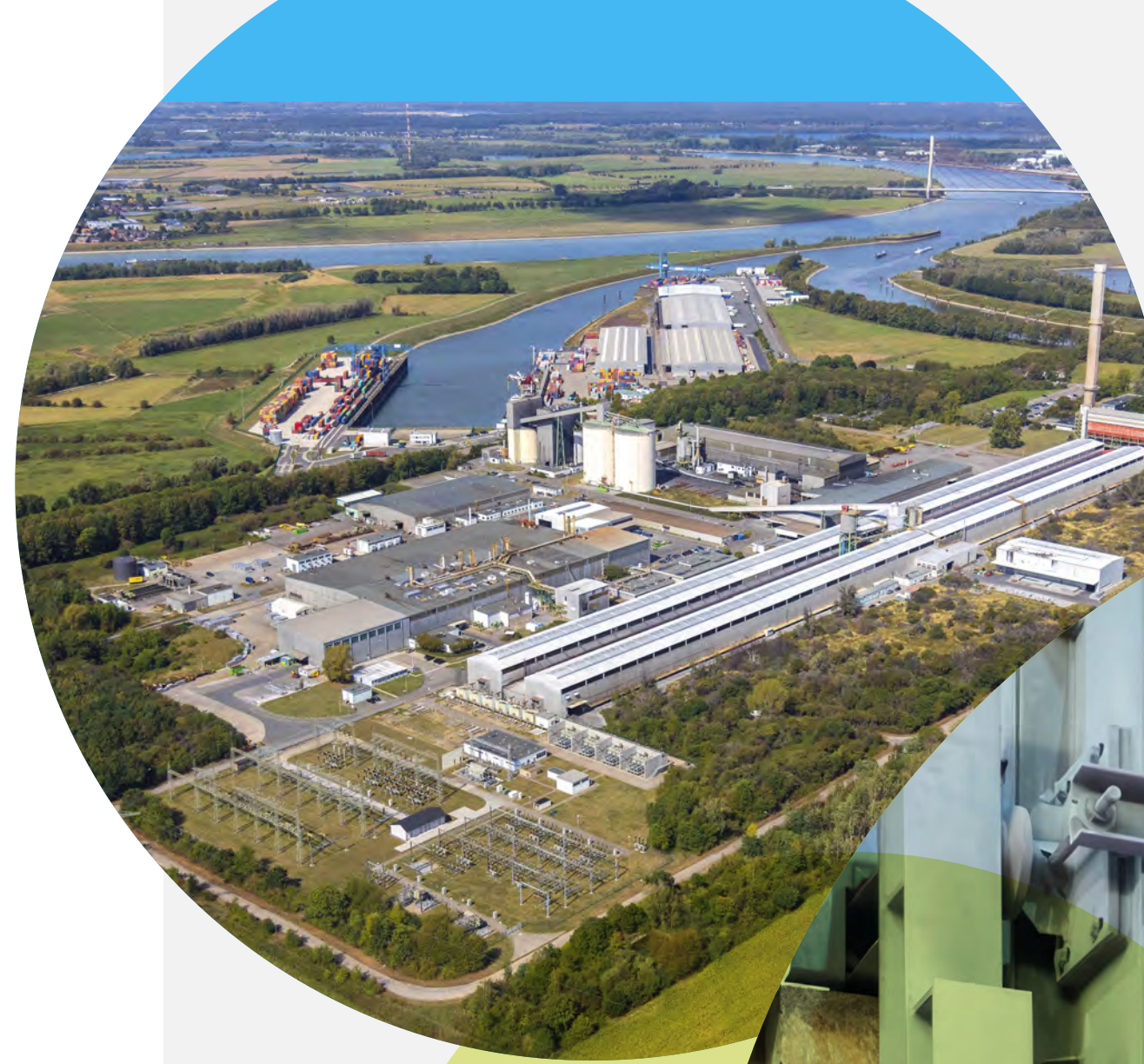
Voerde, Germany, plant
